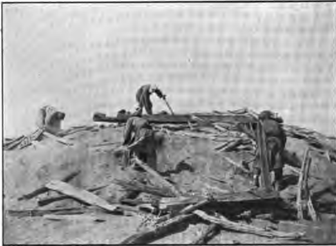
Excavating the Buddhist Temple.
