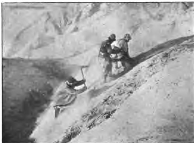
Making a Road over the First Pass.
